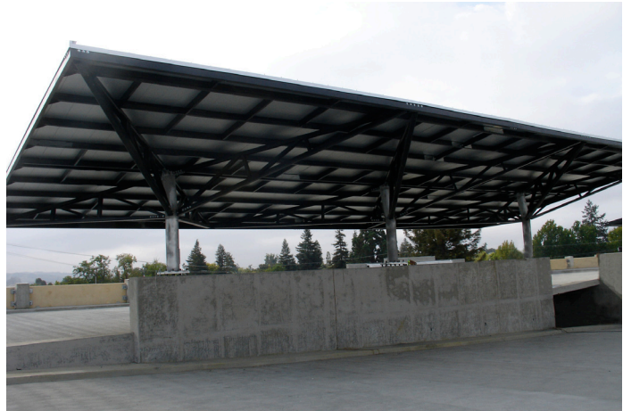
City of Napa Fifth Street Parking Garage Intersection of Fifth and Main Streets, Napa, CA 94559
